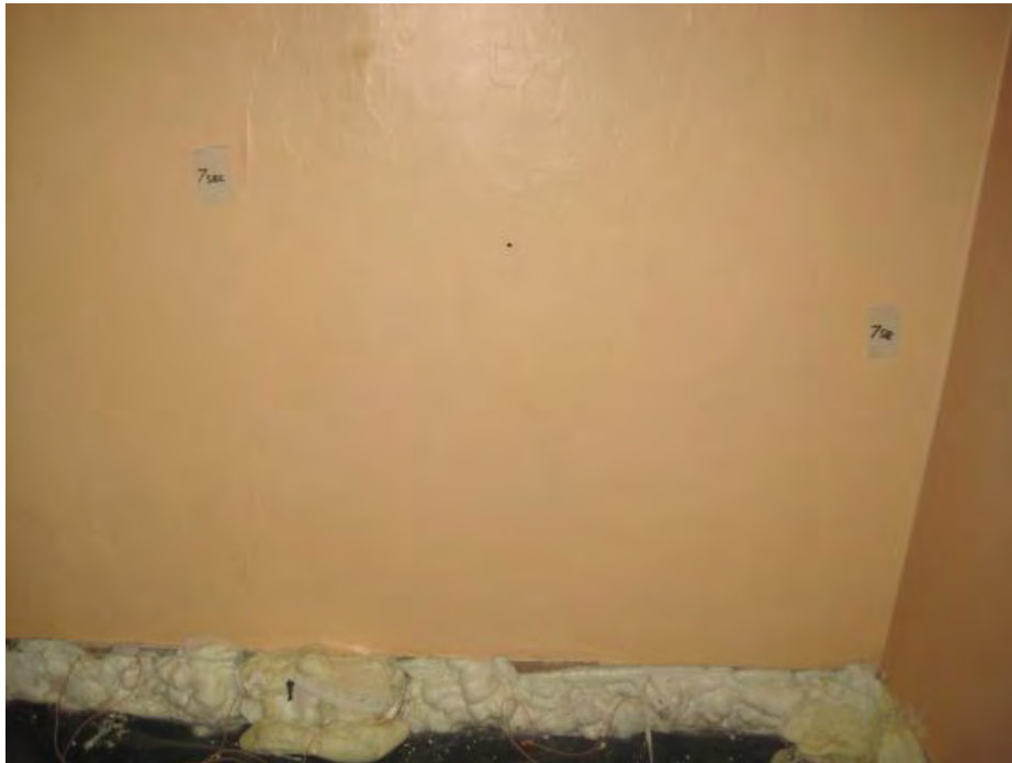
Leak of the foam at the bottom part of the wall
