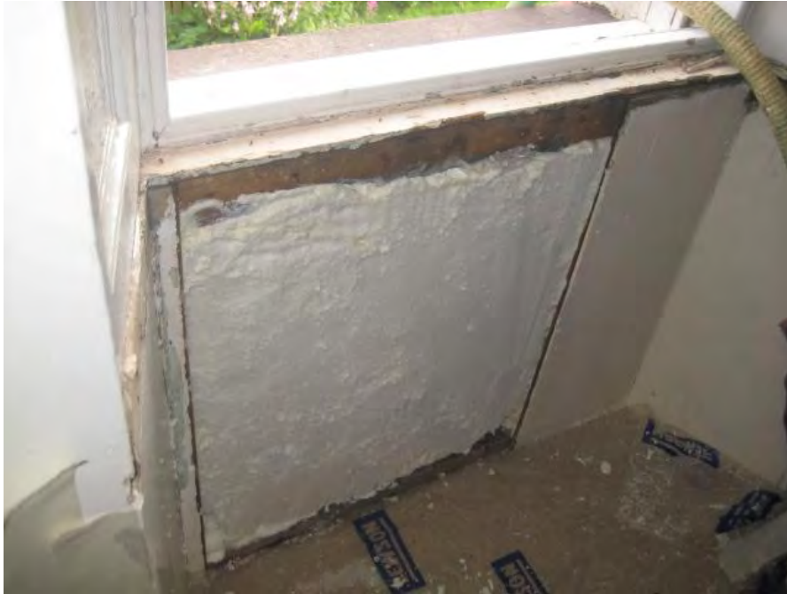
Insulating the wall under the window
