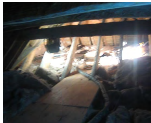
Floor covering and lighting installed for safety and easy access to the loft
