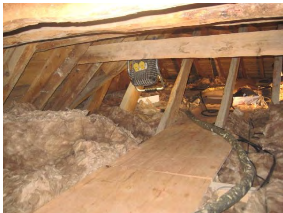
Floor covering and lighting installed for safety and easy access to the loft
