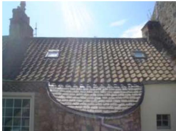
Fig. 11 Back elevation with stepped coping stones above party walls
