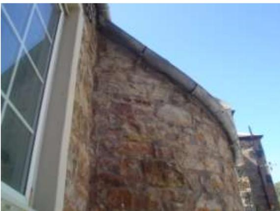
Fig. 05 Curved stair case and bedroom rubble stone walls
