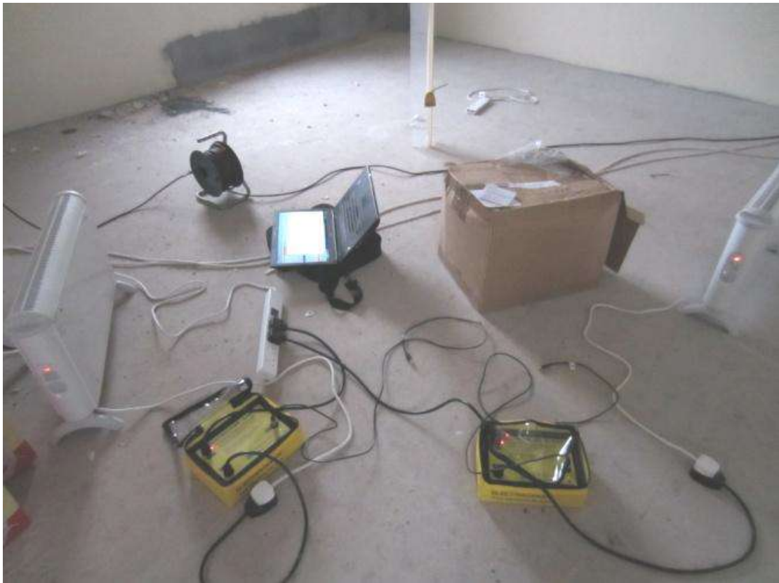
Figure 3. Electrical convector heaters and ElectroCorder Voltage & Current data loggers in Locate room (Photograph from Uist HtT Housing Project 2011-12 Final Report Part 2).
