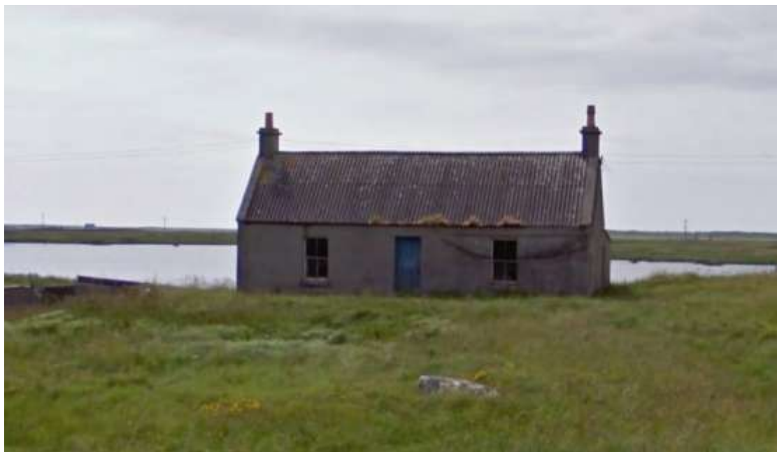
Figure 1. Typical single storey two bedroom stone walled croft house at Daliburgh, South Uist (Photograph from Uist HtT Housing Project 2011-12 Final Report Part 2).
