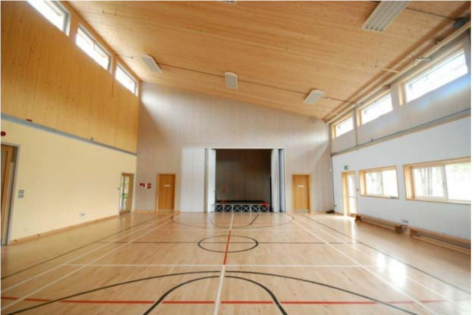
Figure 6. The high clerestorey lights provide the majority of daylight. The low windows face north so there is no glare, and good uniformity of light. The clerestorey lights also open to let hot air escape when needed
