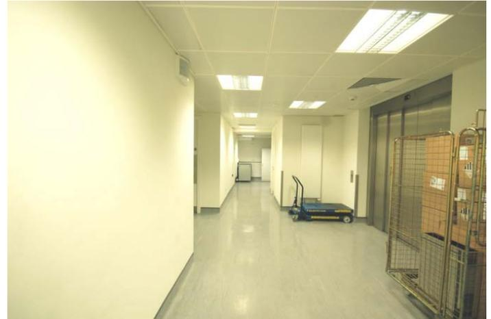
Figure 5. Excessive light levels in a corridor. Half the lights would still exceed minimum standards.
