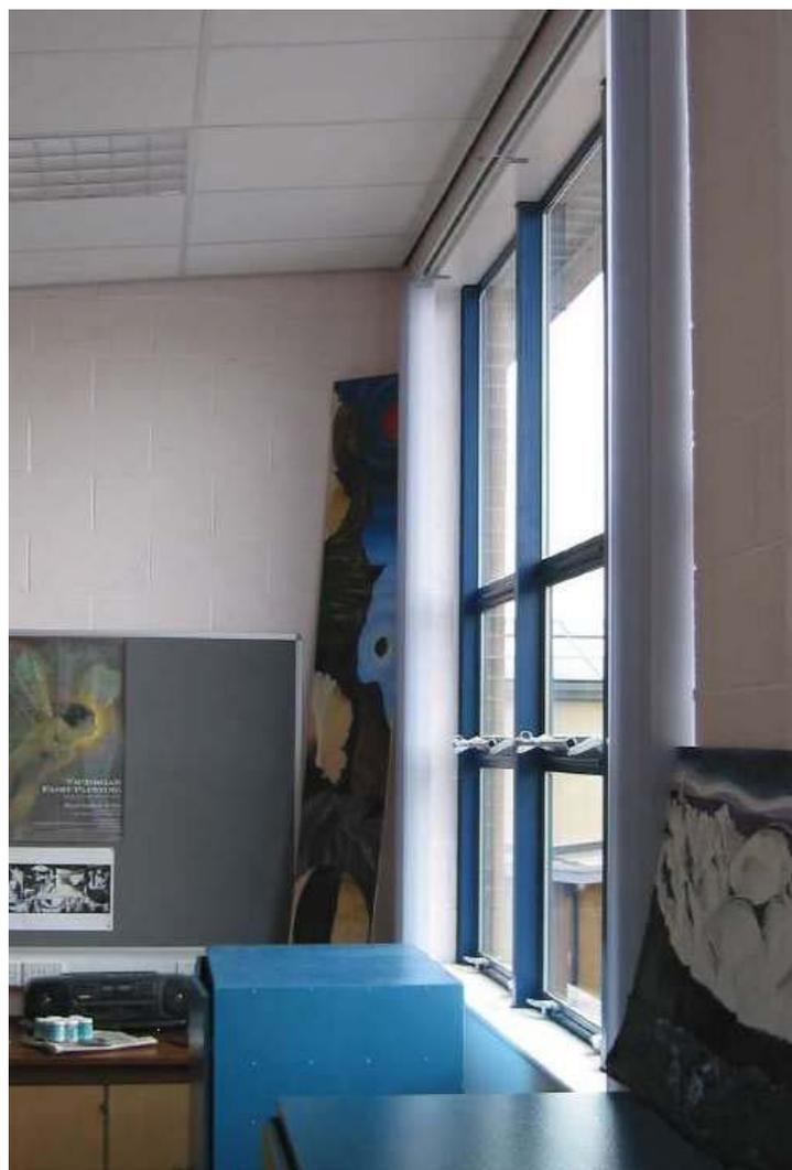
Figure 1. Hot air trapped at the ceiling due to poor window design, only the middle and bottom panes can be opened preventing hot air from escaping
