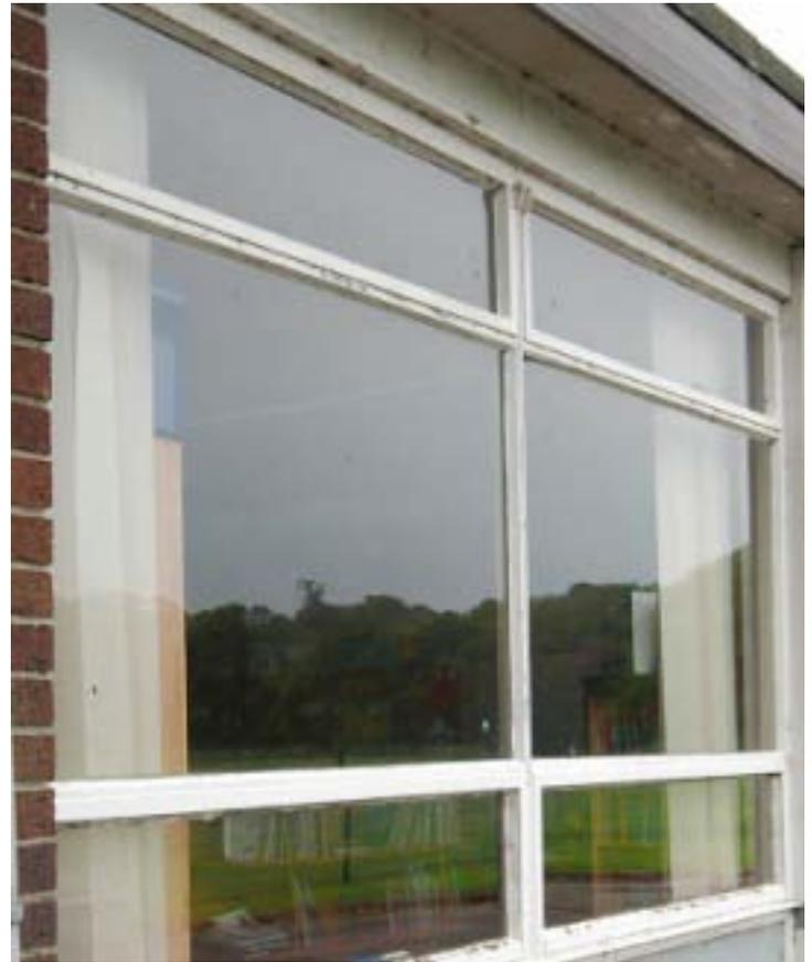
Figure 1. About 15% of the window is obscured by the blinds when they are open. The blinds will also hinder the ventilation
