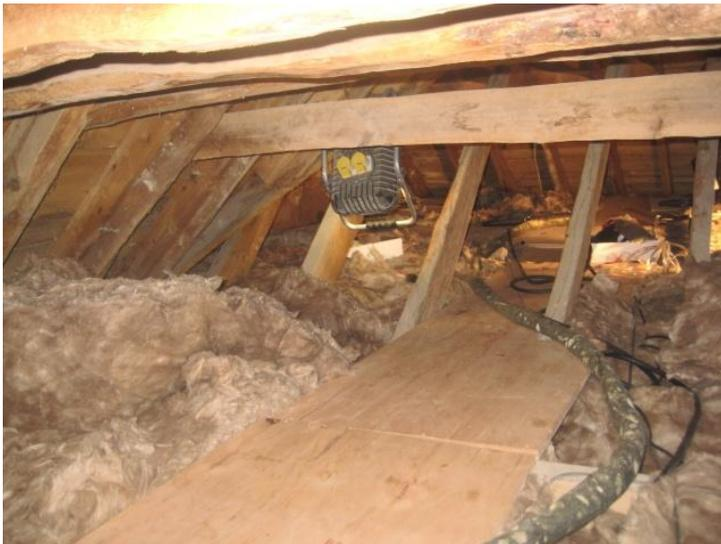
Picture 3. Floor covering and lighting installed for safety and easy access to the loft
