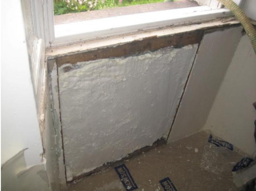
Picture 8. Insulating the wall below the window
