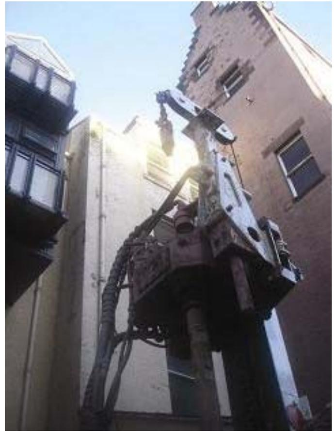
The drilling rig onsite for the ground source heat pumps bore holes with the existing south elevation prior to the installation of the sunspaces
