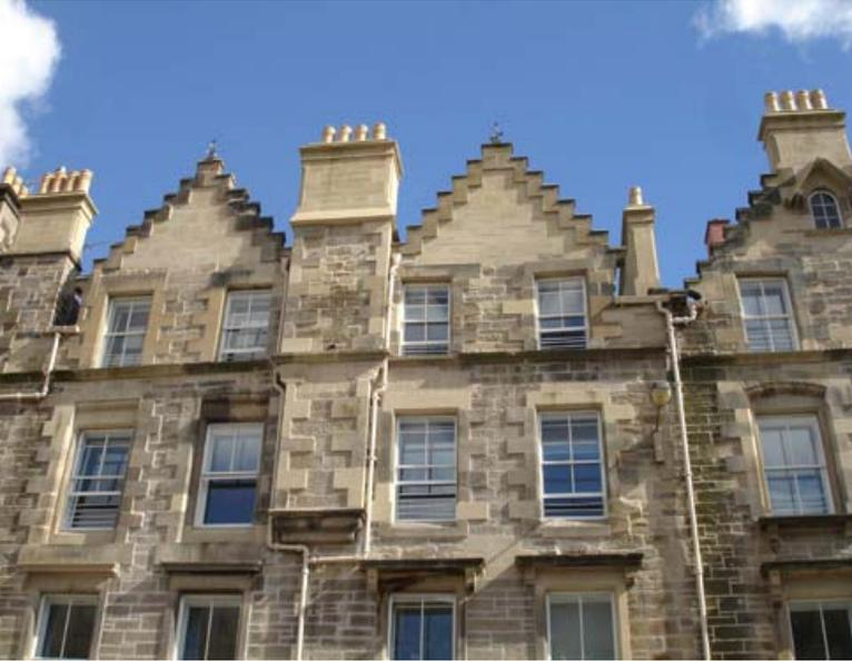
The windows also posed a significant problem, being original sash and case single glazed units. Due to the building's location within the Edinburgh World Heritage site, it was not possible to replace the windows with double or triple glazing, so we opted for secondary glazing, which had to meet EWHT's conservation requirements, to help reduce the heat loss from the flats.
