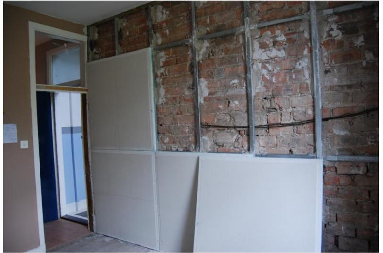
Fig.5 Insulating board being applied to new metal strapping
