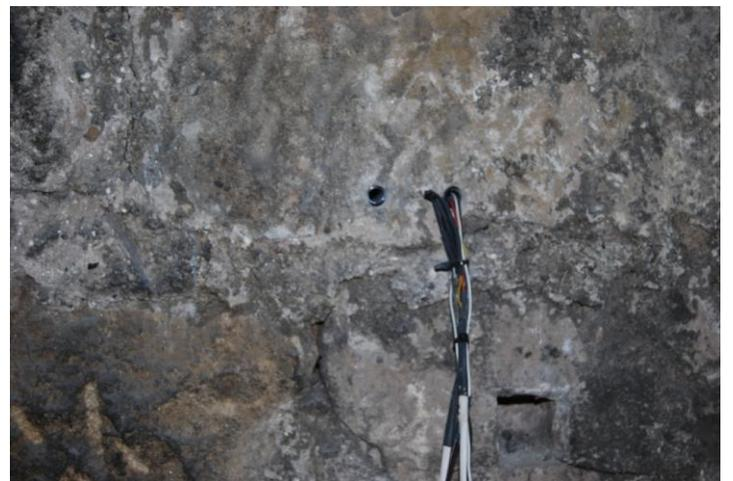
Fig.6 Monitoring equipment was installed to measure both the thermal performance of the wall and the build up of moisture within the wall
