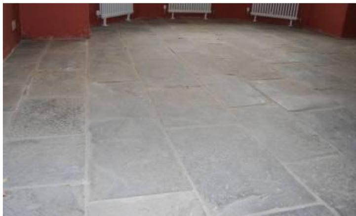
Fig.10 Hemp and lime concrete insulated floor at Blackburn house currently being tested
