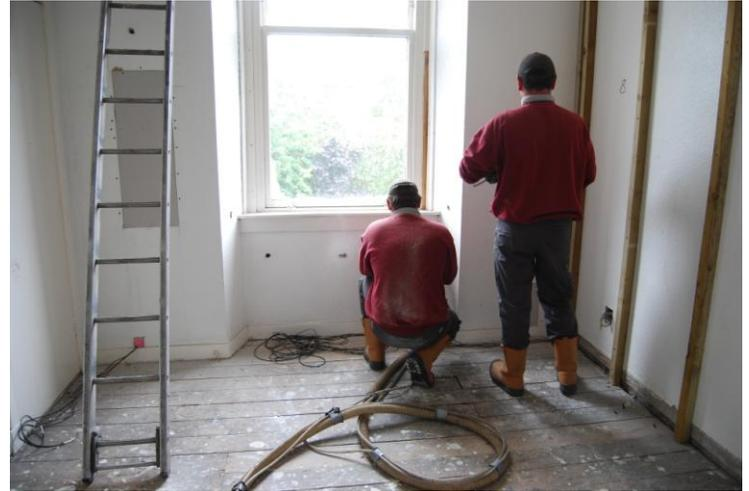
Fig.8 Application of bonded polystyrene bead insulation into cavity between plasterboard and wall
