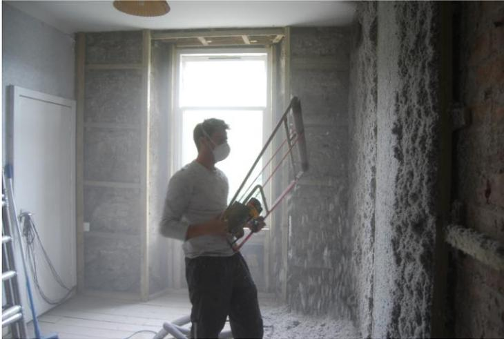
Fig.7 Finishing blown cellulose insulation applied wet directly onto wall
