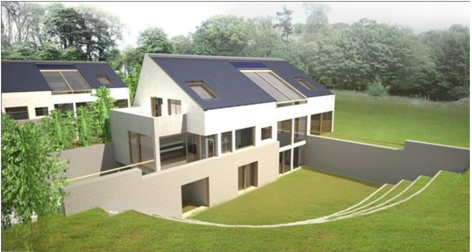
Figure 1: South-west Façade Image of the Z-en House: ROBERTRYAN Homes (Source: MEARU, Mackintosh School of Architecture)
